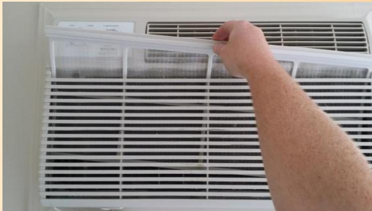
Once removed you can use a small brush or paper towel to brush the dust off. After most of the dust is off, give it a good rinse. If there is any discoloration to the screen rub a small amount of dawn dish soap on and let it sit for 5 minutes before rinsing again.
